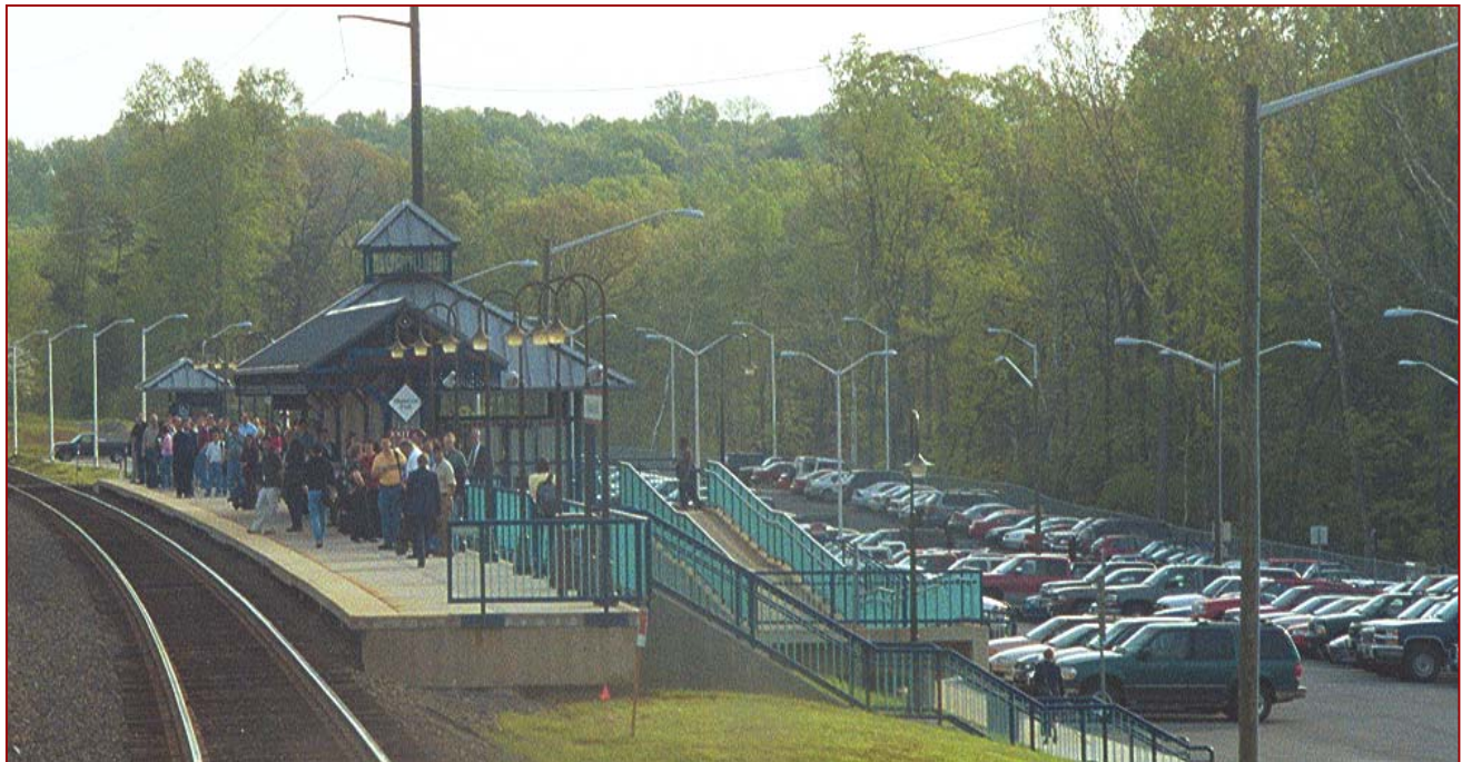
Rail station with Park and Ride Lot
